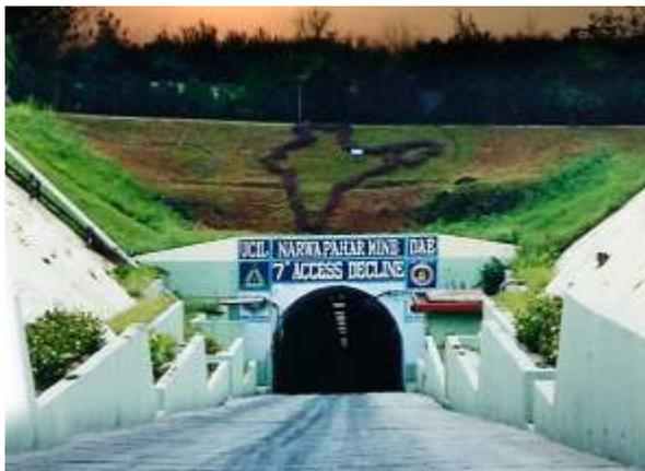
Narwapahar mine in operation since 1995, is accessed by a 355 meter deep vertical shaft and a 7° access decline from the surface. The layout of the mines facilitated deployment of trackless equipment. The production capacity of the mine is being augmented to 1500 tonnes per day.
